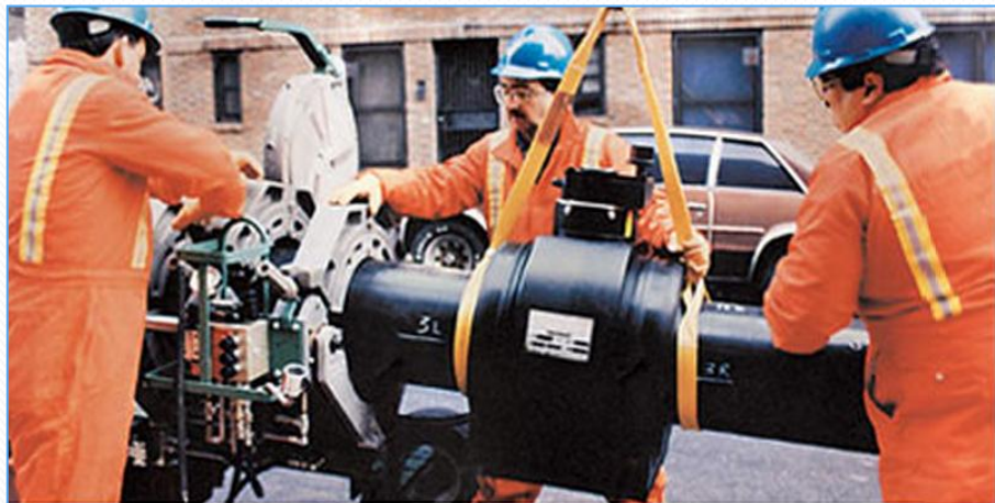
12" Poly-Gas ® valve fusion operation
